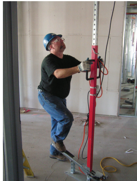
Figure 3. New foot-lever drill press with the same drill saddle on top (not visible) as in Figure 2. The inner column is first lifted to a height for drilling and locked with the gravity pin just above the black handles. Then the foot lever is used to advance the drill during drilling.
