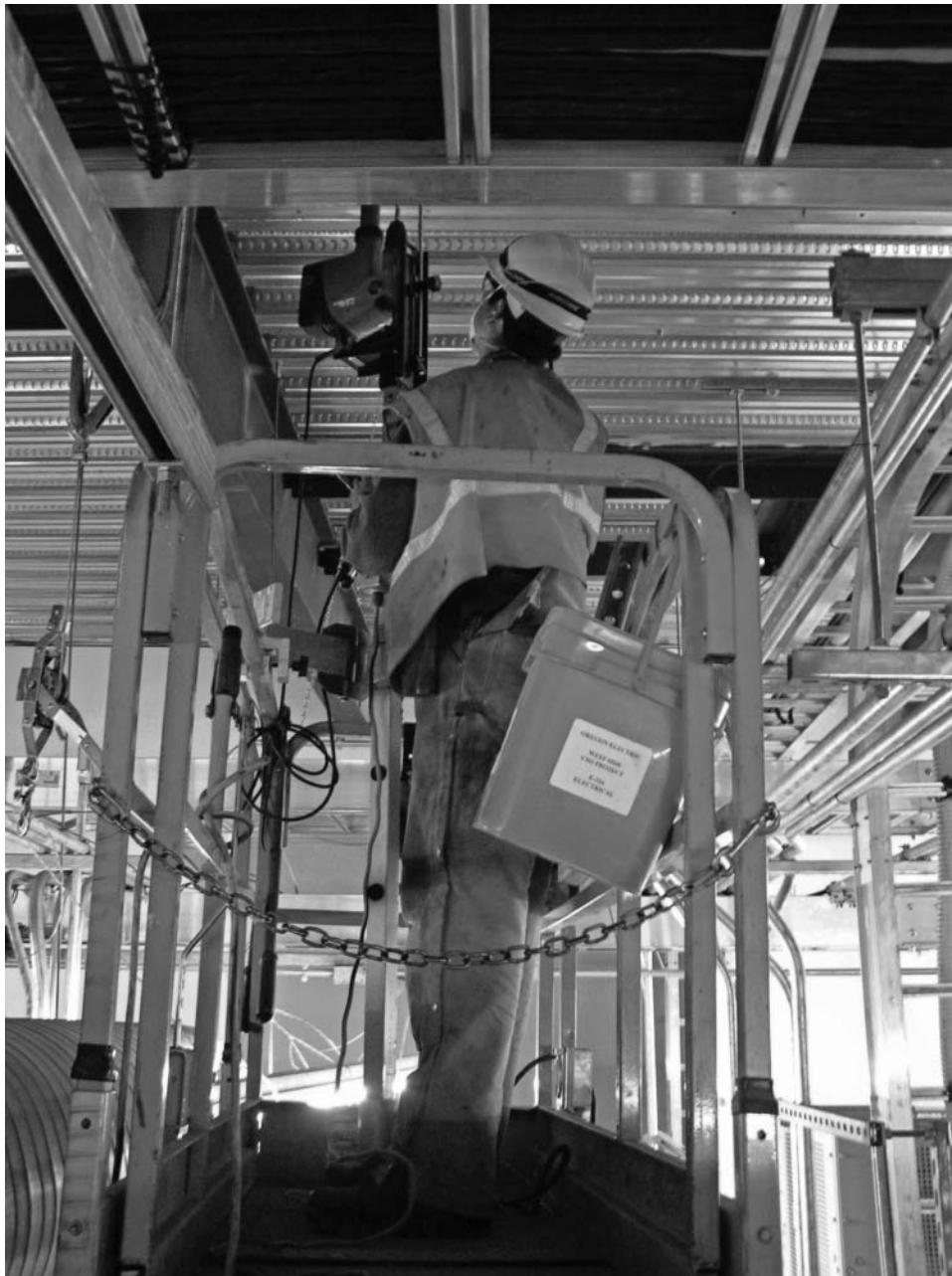
FIGURE 4. The intervention design used in a scissor lift. The wheeled base is replaced with a round plastic disk.
