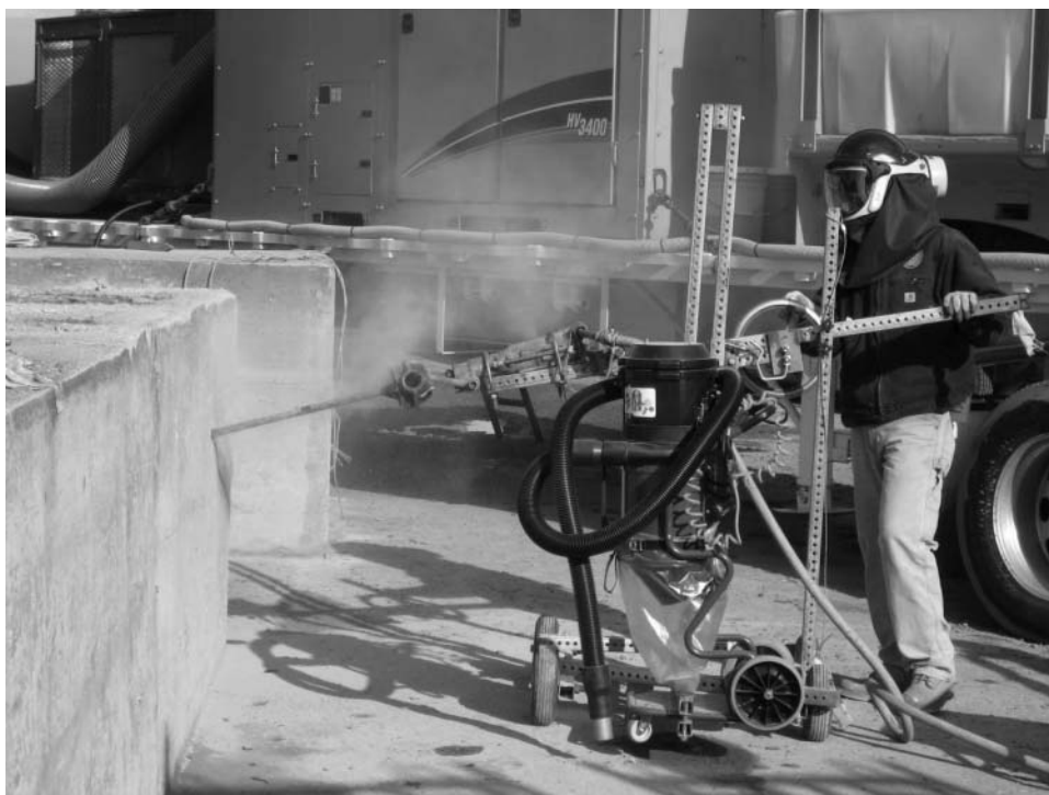
FIGURE 2. Pneumatic drill with support jig (vacuum is not used).
